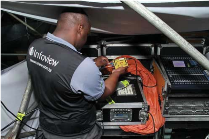
Infoview technician installs CDH 1813 SDI to HDMI converters
